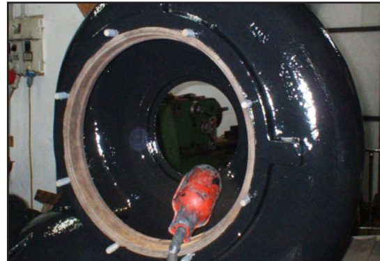
ARC coated surface after proper surface preparation
